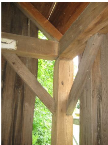
Classic post and beam construction at the West Cemetery Hearse House.
