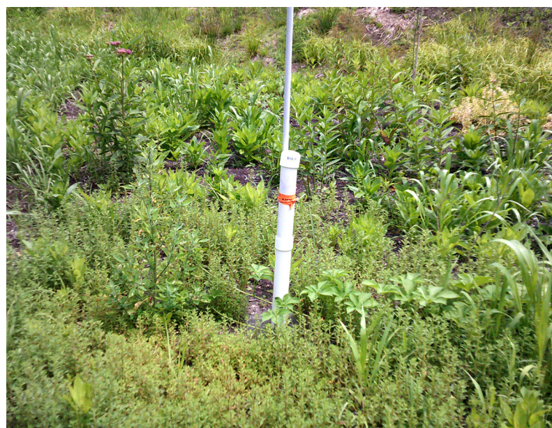
Figure 14 Monitoring piezometer located in wetland replacement area
