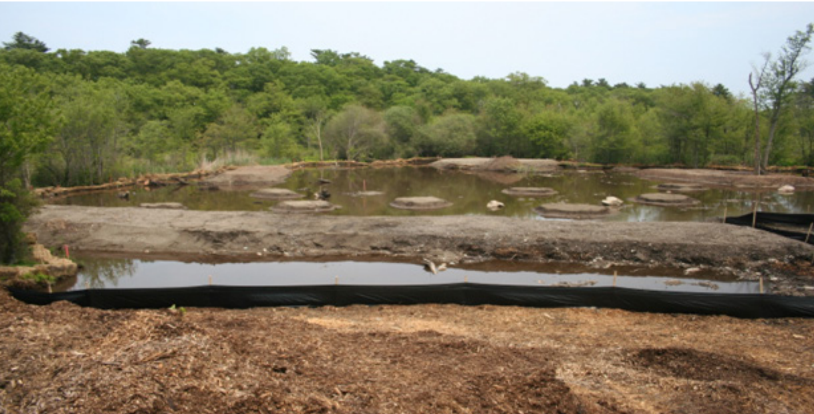
Figure 1 Example of a wetland replacement area in progress
