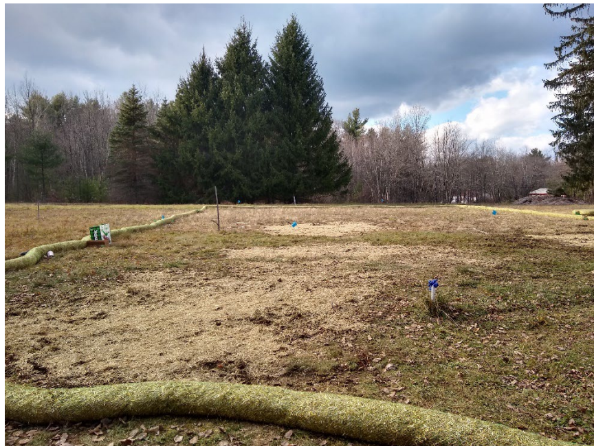
Photo 8 Test pits covered with native material and straw/hay..
