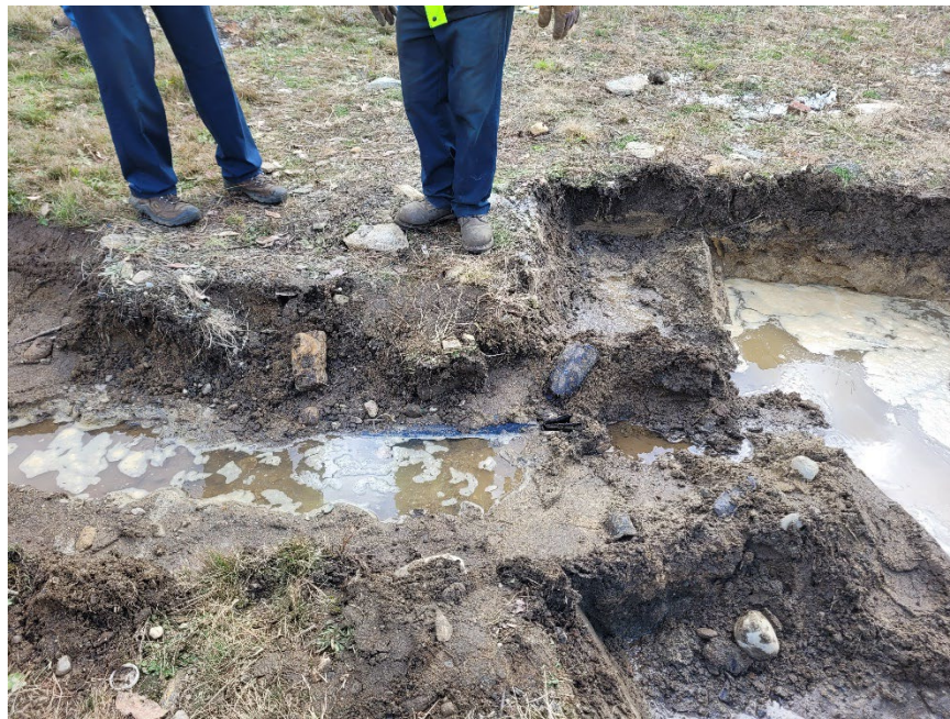
Photo 6 Drainpipe in center of photo. Beginning of drainpipe in right portion of photo. Test pit 1.
