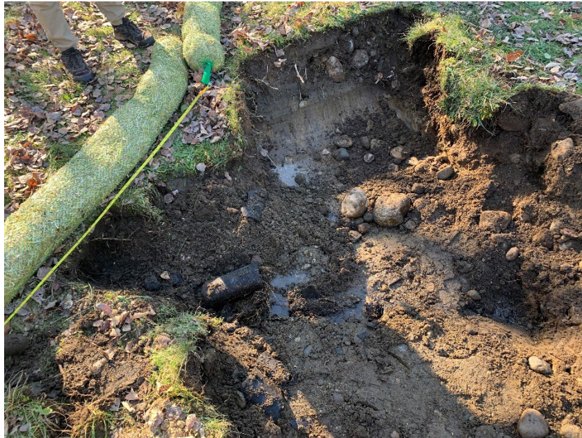
Photo 3 Drainpipe and eastern boundary of work area. Test pit 2.
