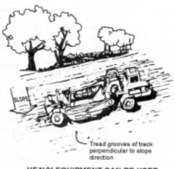
HEAVY EQUIPMENT CAN BE USED TO MECHANICALLY SCARIFY SLOPES
