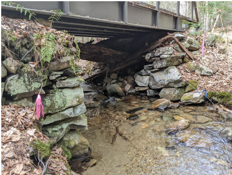
Photo 6: 3/23/22 – View of the stream channel and abutments (from downstream).
