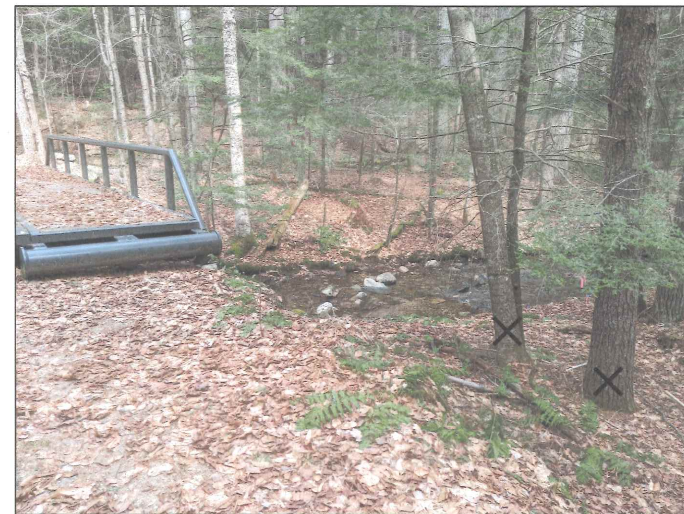
⑥ SOUTHERN BRIDGE APPROACH (LOOKING NE)
