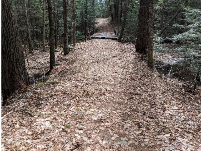
Photo 1: 3/23/22 – View southerly along Cornwell Road.
