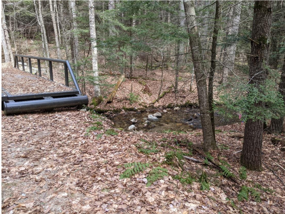
Photo 9: 3/23/22 – View from the south of Camel Brook Crossing.
