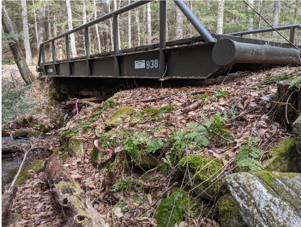
Photo 3: 3/23/22 – View from the southwest looking at existing portable bridge.
