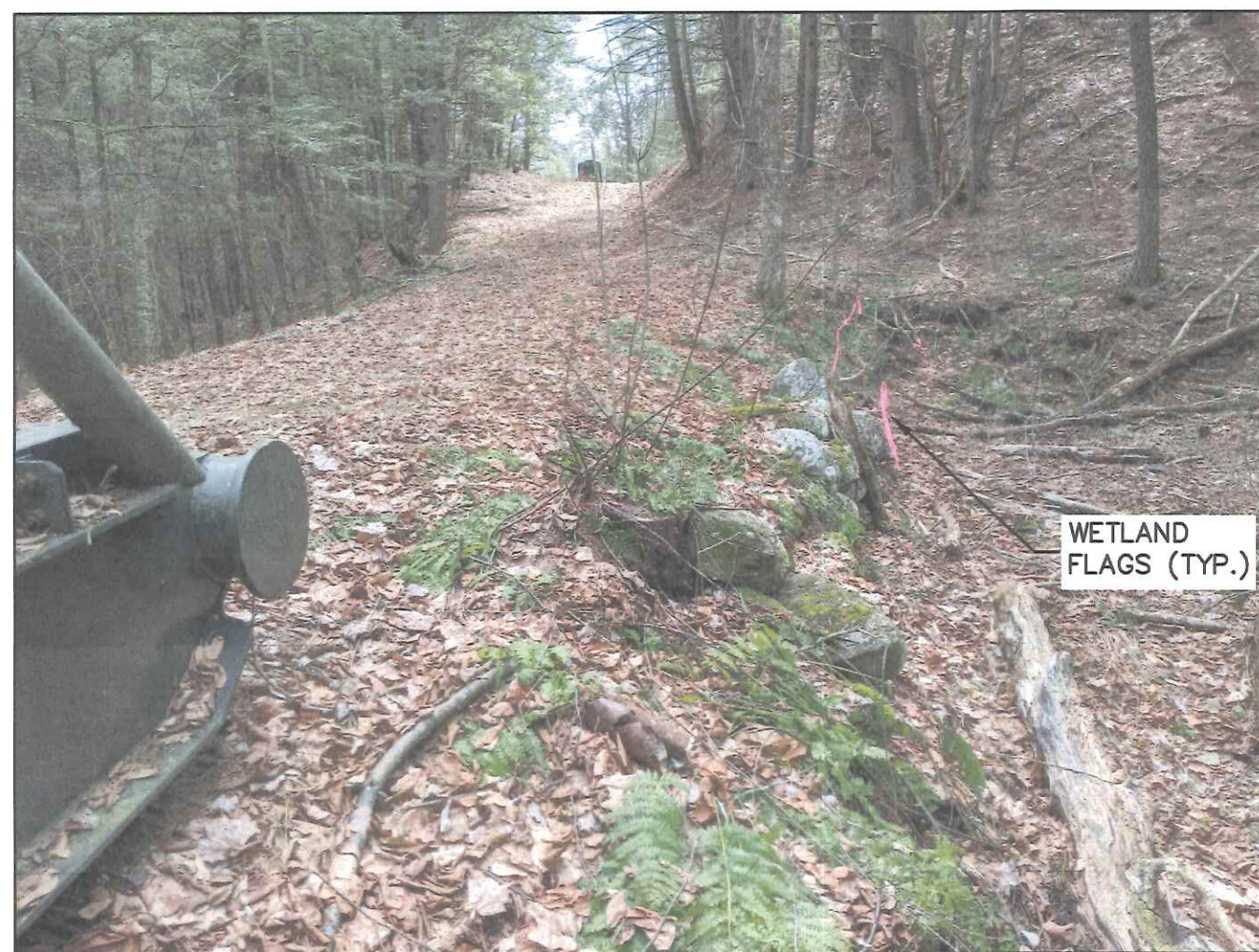
⑤ SOUTHWEST BRIDGE CORNER (LOOKING S)
