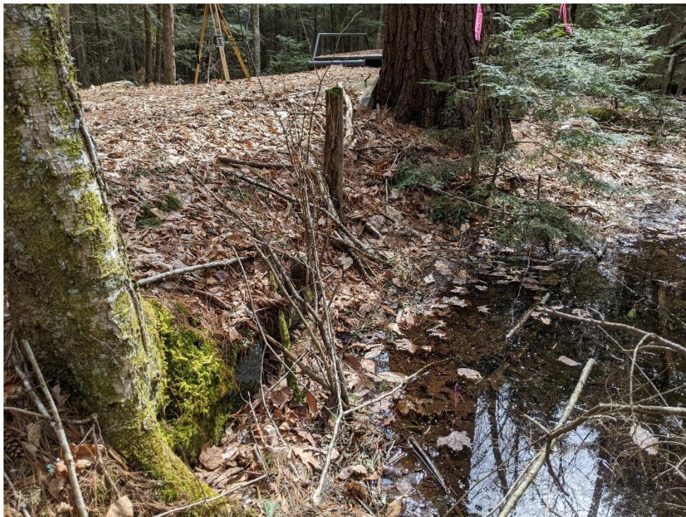
Photo 12: 3/23/22 – Upstream of the apparent drainage structure (north of Camel Brook).
