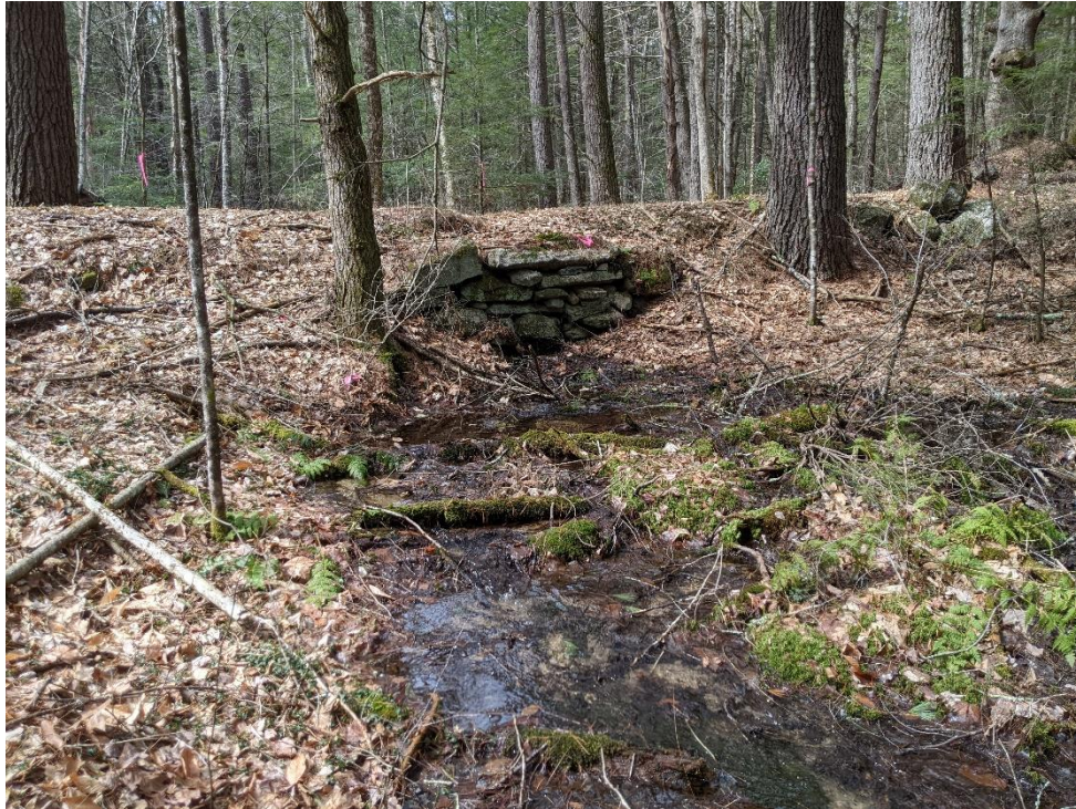
Photo 11: 3/23/22 – Headwall and drainage structure to the north of Camel Brook (downstream).
