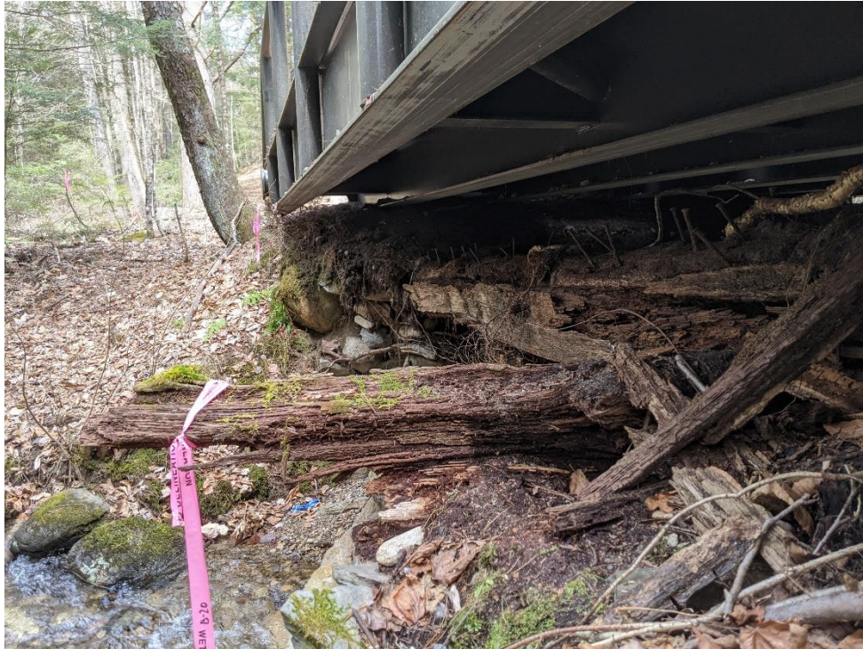
Photo 5: 3/23/22 – Former timber bridge under portable bridge (from upstream).
