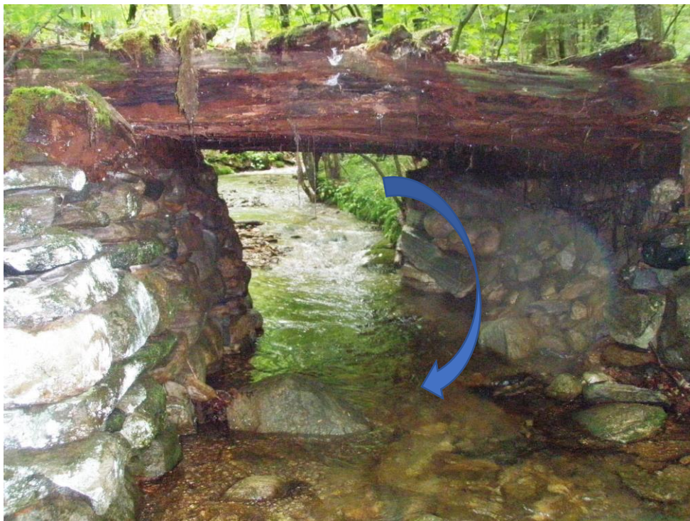
Photo 4: 6/25/2009 – View from downstream from the original wooden bridge.
