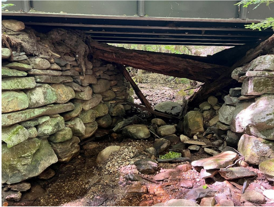
Photo 13: 9/3/22 – View from the east, under the bridge.
