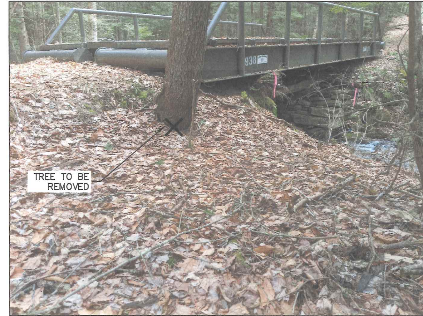
② NORTHWEST BRIDGE CORNER (LOOKING SE)
