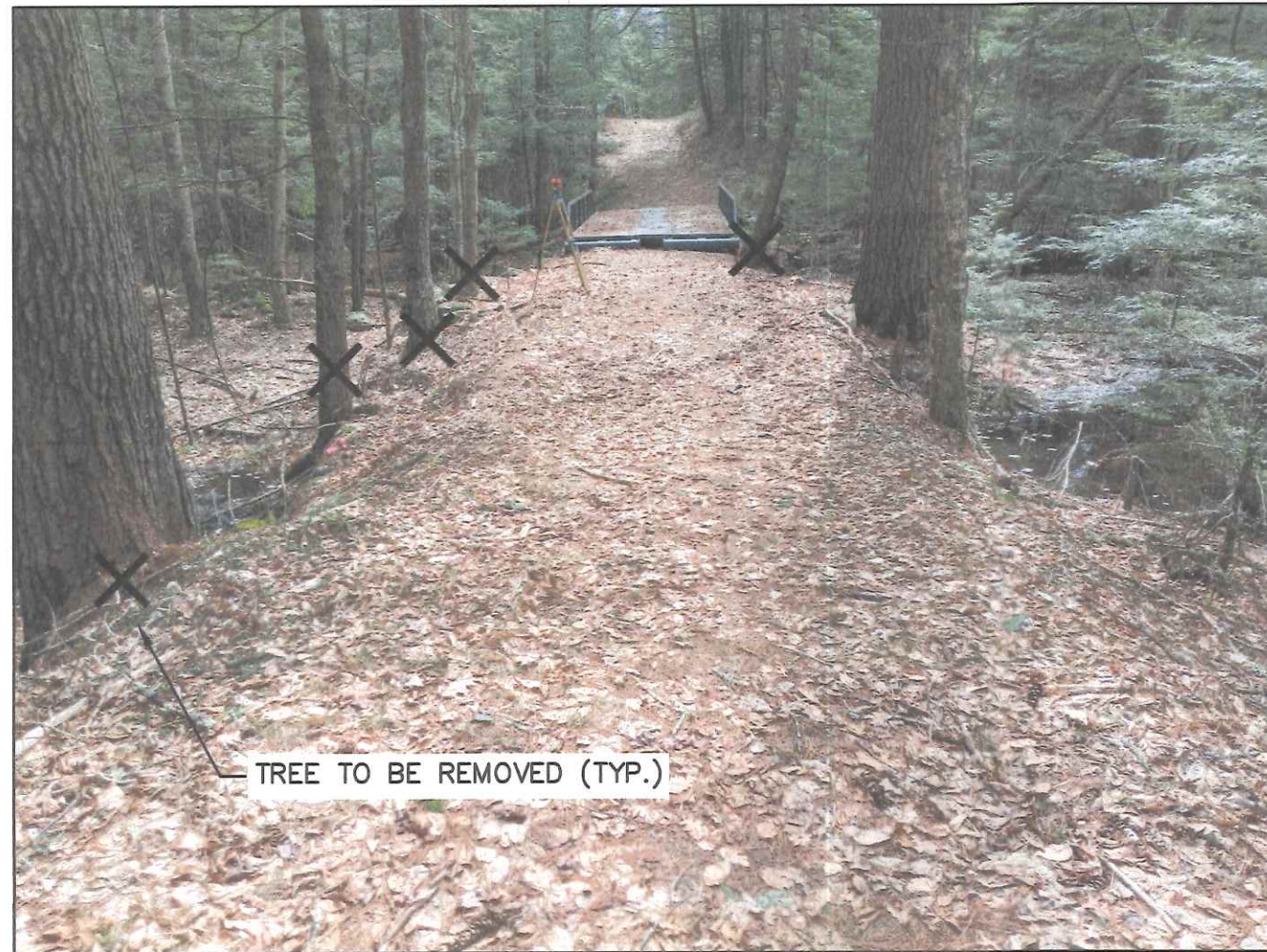
① NORTHERN BRIDGE APPROACH (LOOKING S)
