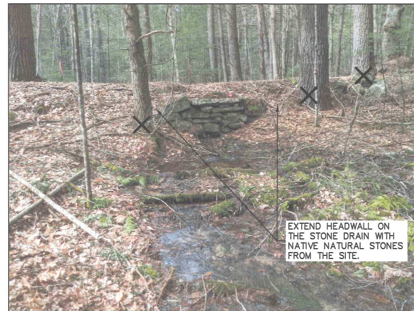
⑩ NORTHERN APPROACH CULVERT UPSTREAM (LOOKING W)
