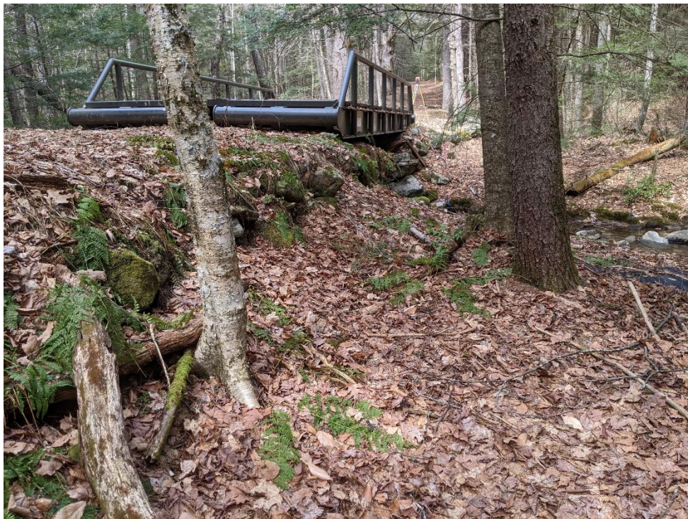
Photo 10: 3/23/22 – Southeastern shoulder and wall.
