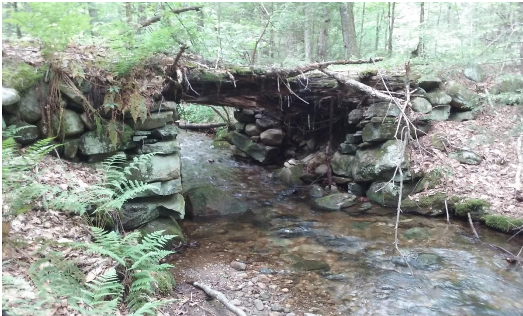
Photo 2: 6/09/2017 – View of wooden bridge crossing at Cornwell Road.
