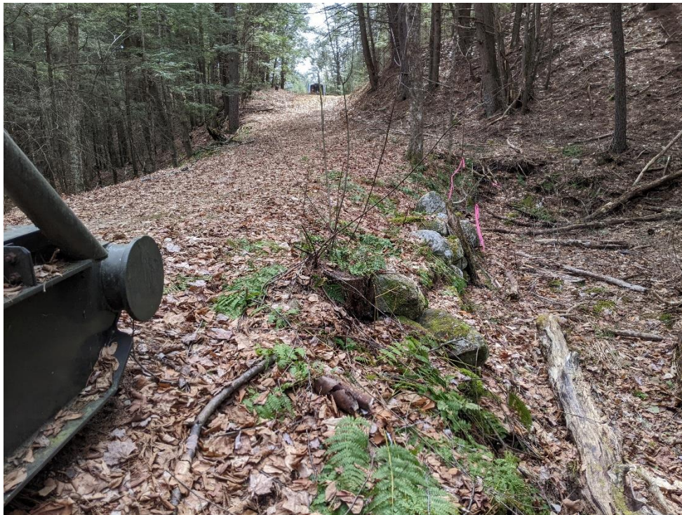
Photo 4: 3/23/22 – View of the southern approach from the existing bridge.
