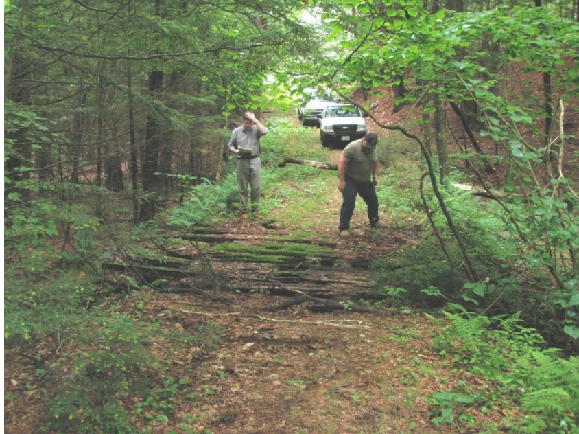
Photo 1: 6/25/2009 – View of wooden bridge deck along Cornwell Road.
