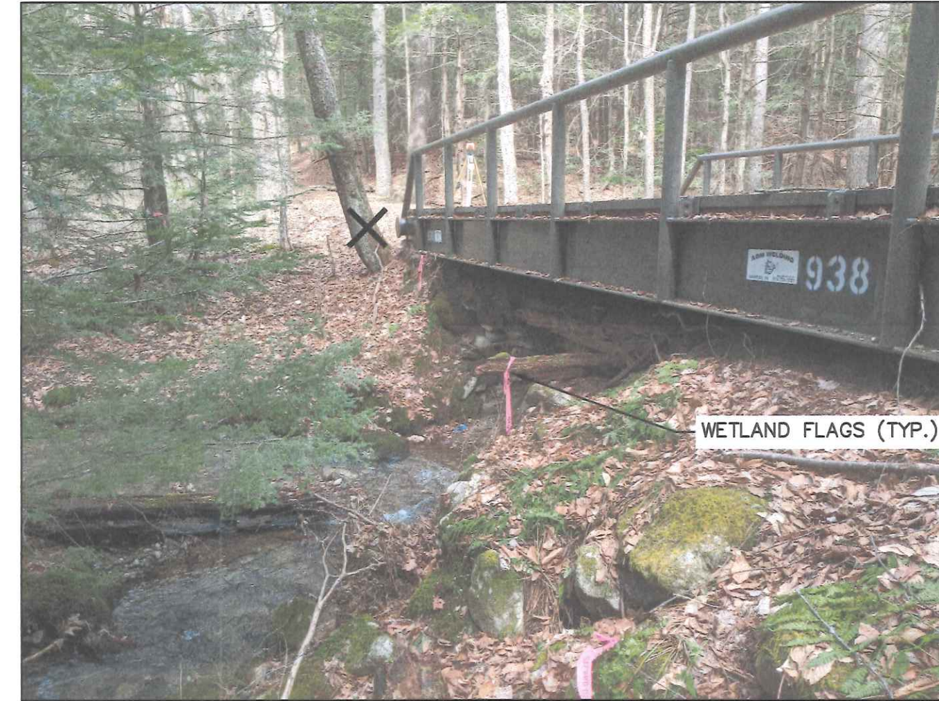
③ SOUTHWEST BRIDGE CORNER (LOOKING NE)
