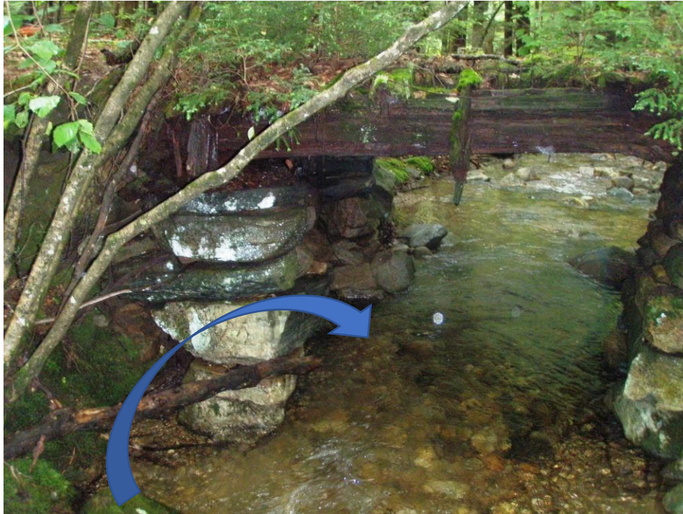
Photo 3: 6/25/2009 – View from upstream approach to crossing at Cornwell Road bridge.
