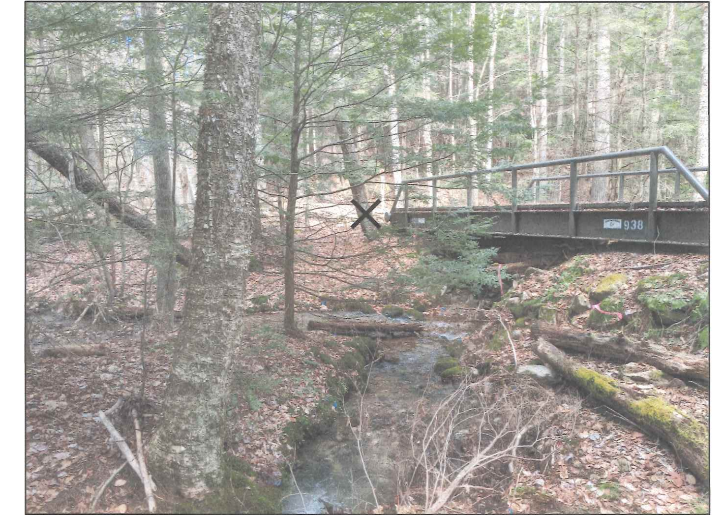
④ UPSTREAM BRIDGE VIEW (LOOKING E)
