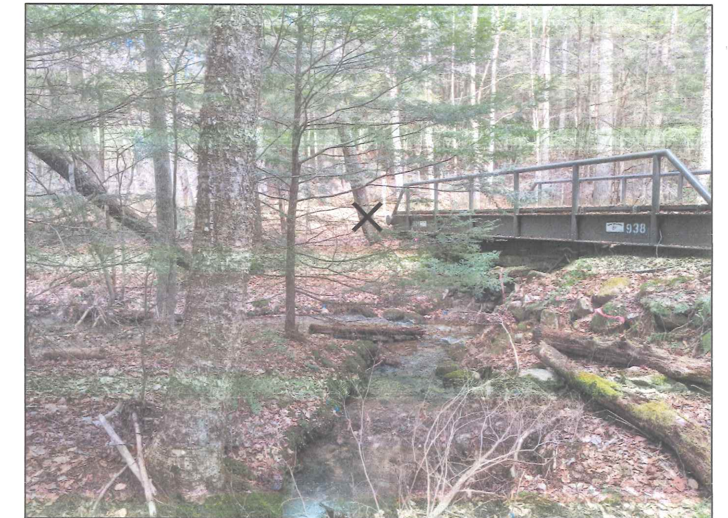
④ UPSTREAM BRIDGE VIEW (LOOKING E)
