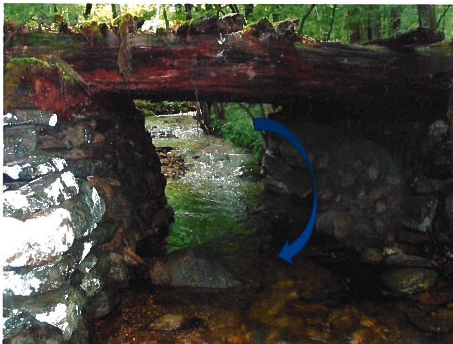
Photo 4: 6/25/2009 – View from downstream from the original wooden bridge.
