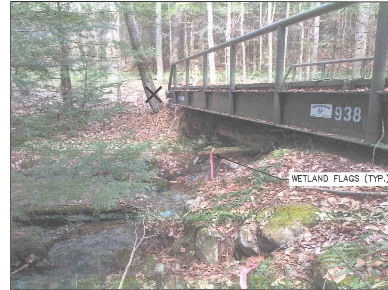
③ SOUTHWEST BRIDGE CORNER (LOOKING NE)
