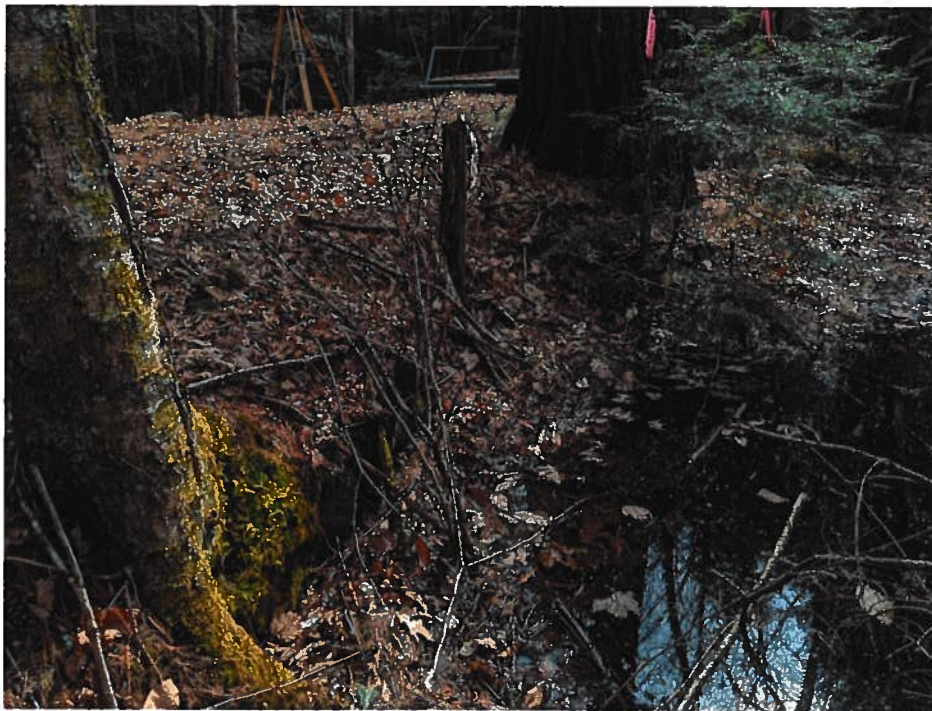
Photo 12: 3/23/22 – Upstream of the apparent drainage structure (north of Camel Brook).
