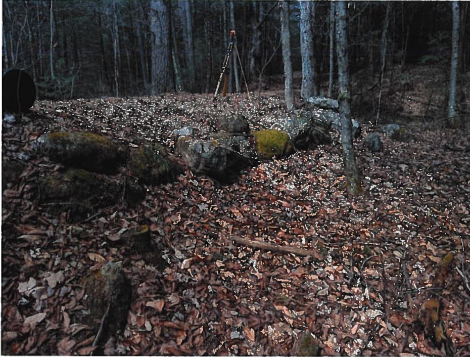
Photo 7: 3/23/22 – View of the shoulder on the north approach.
