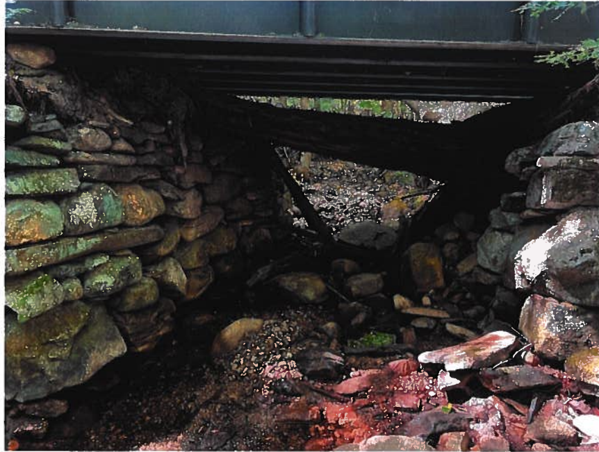
Photo 13: 9/3/22 – View from the east, under the bridge.
