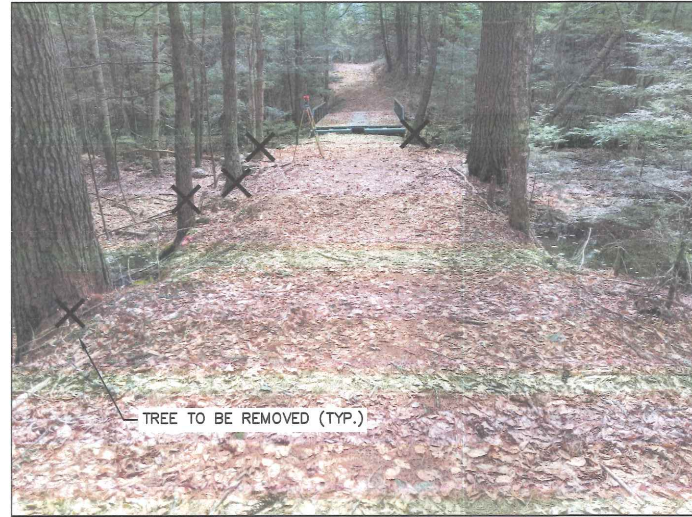
① NORTHERN BRIDGE APPROACH (LOOKING S)
