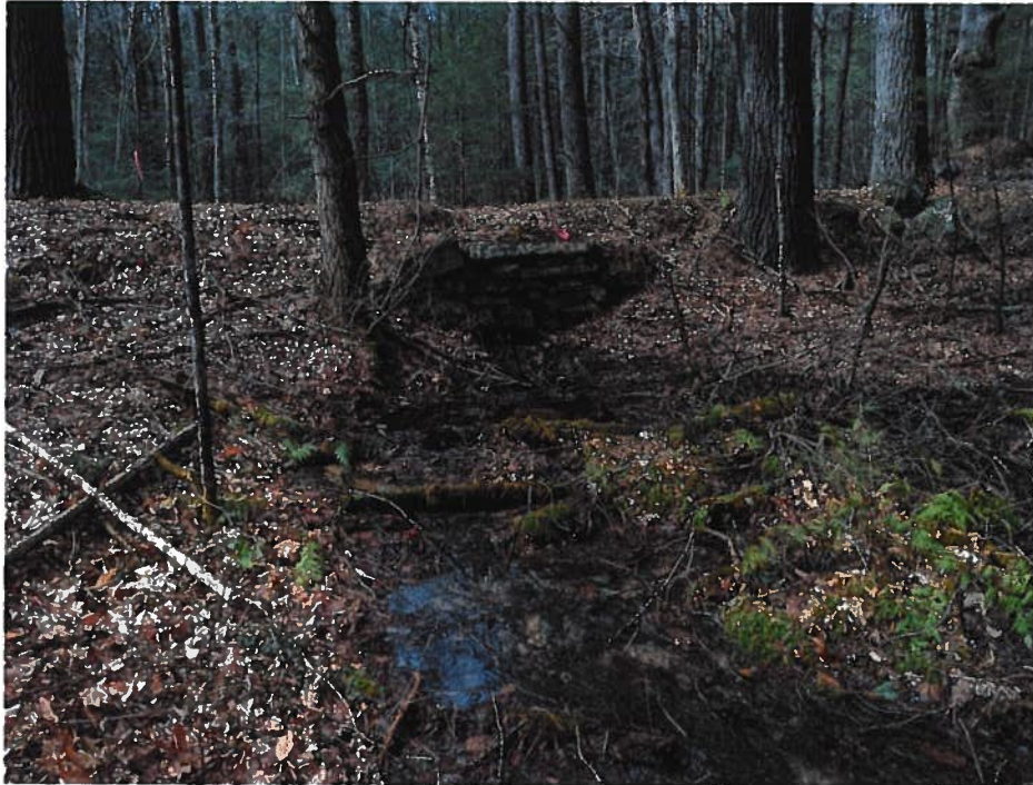
Photo 11: 3/23/22 – Headwall and drainage structure to the north of Camel Brook (downstream).
