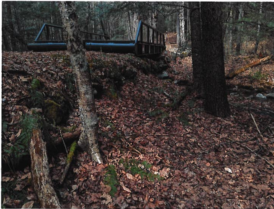
Photo 10: 3/23/22 – Southeastern shoulder and wall.
