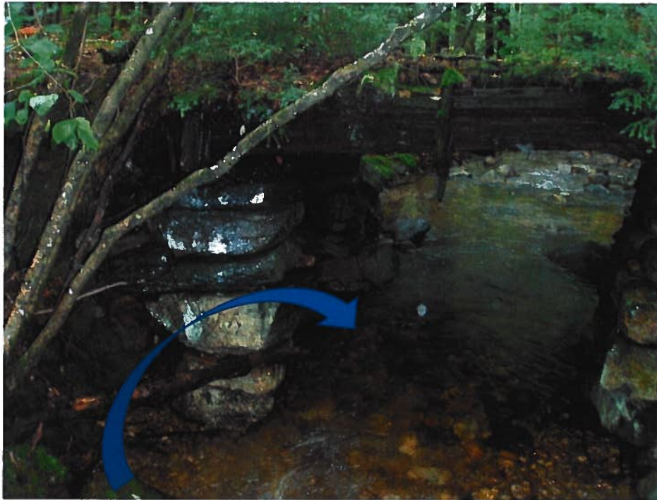
Photo 3: 6/25/2009 – View from upstream approach to crossing at Cornwell Road bridge.
