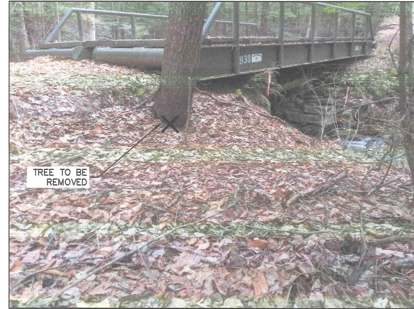
② NORTHWEST BRIDGE CORNER (LOOKING SE)
