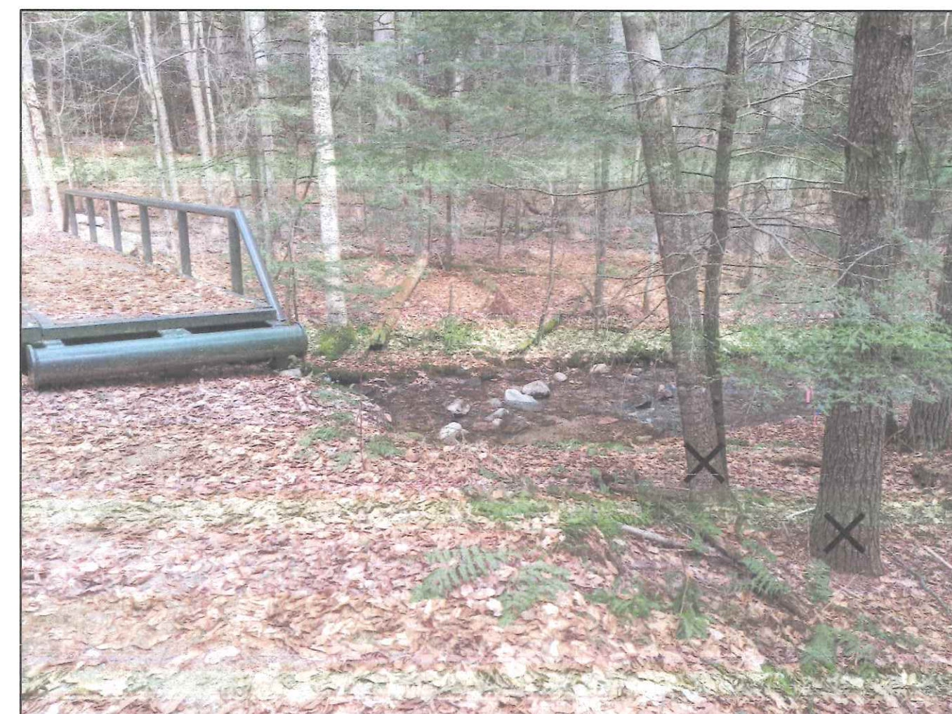
⑥ SOUTHERN BRIDGE APPROACH (LOOKING NE)
