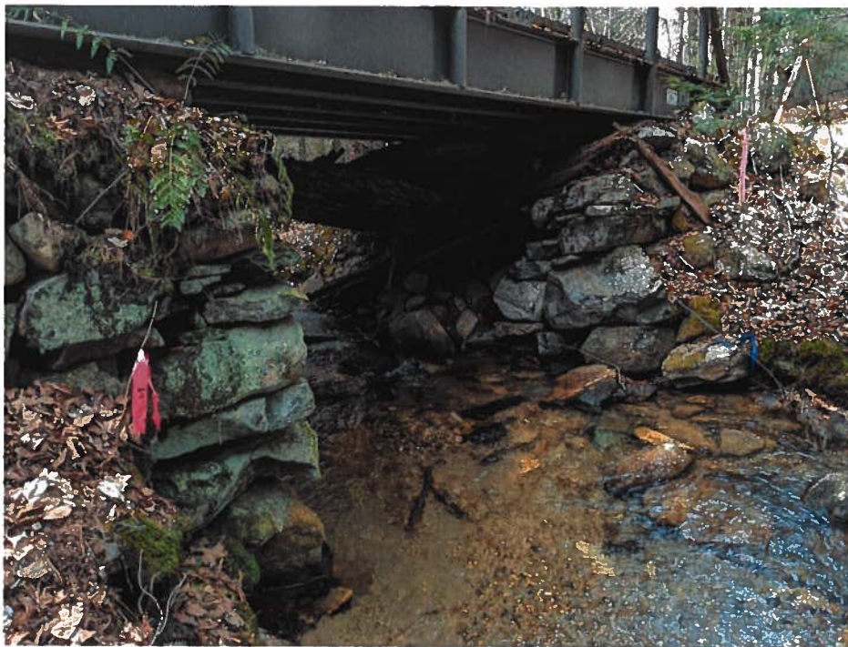
Photo 6: 3/23/22 – View of the stream channel and abutments (from downstream).
