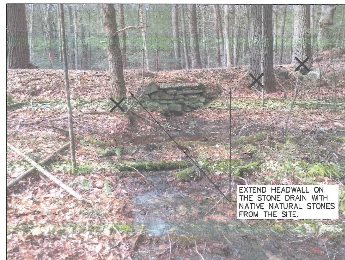
⑩ NORTHERN APPROACH CULVERT UPSTREAM (LOOKING W)
