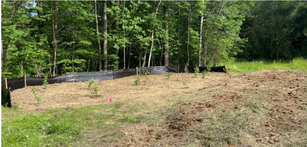
Photo 10 BVW 2 post fill removal and wetland restoration (6/22/23).
