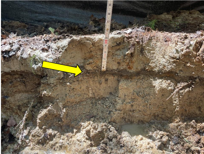
Photo 3 View of the western-most extent of Trench 1 within BVW 3, directly adjacent to the silt fence. The darker horizon was observed at a depth of 5 inches at the toe of slope. This darker horizon may indicate buried topsoil and is indicated with the yellow arrow (6/22/23).
