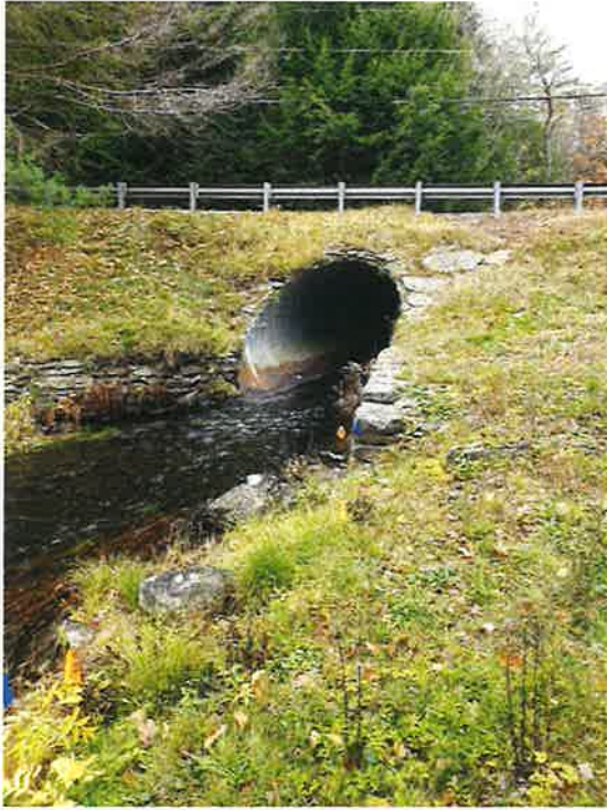
Figure 2. Upstream view of existing culvert
