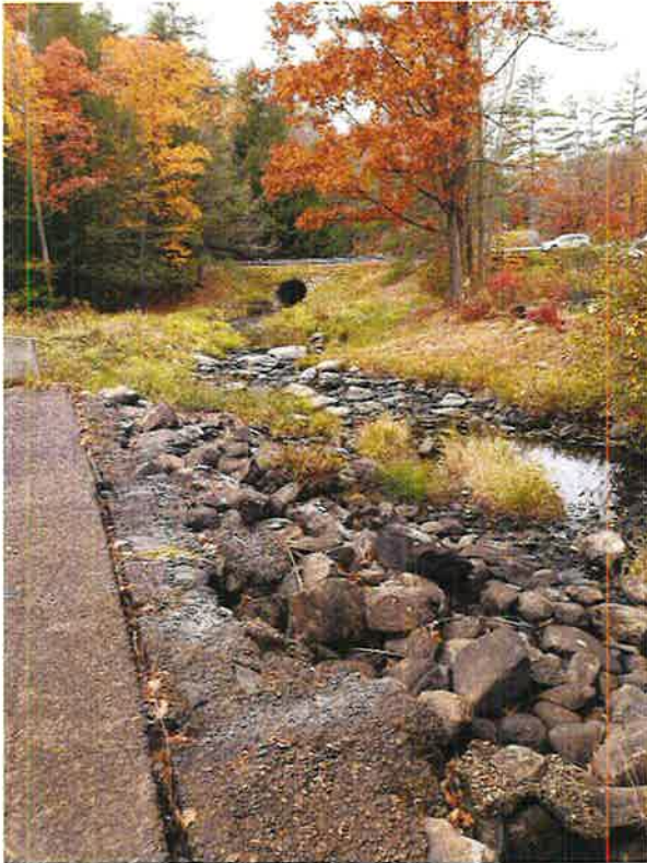
Figure 5: Photo of upstream condition
