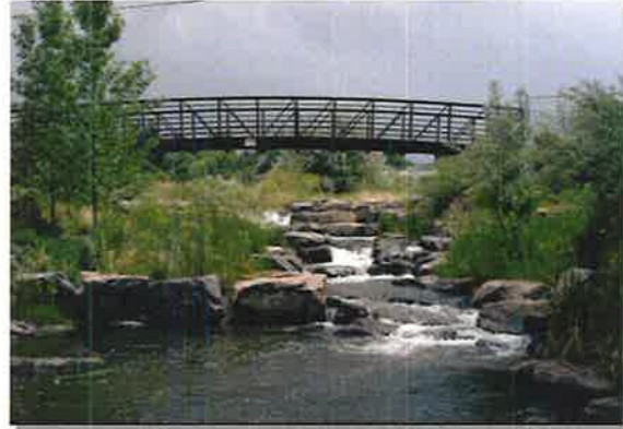
Photograph 9-1. This grouted boulder drop structure exemplifies the opportunity available for creating an attractive urban hydraulic setting for a riparian corridor.
