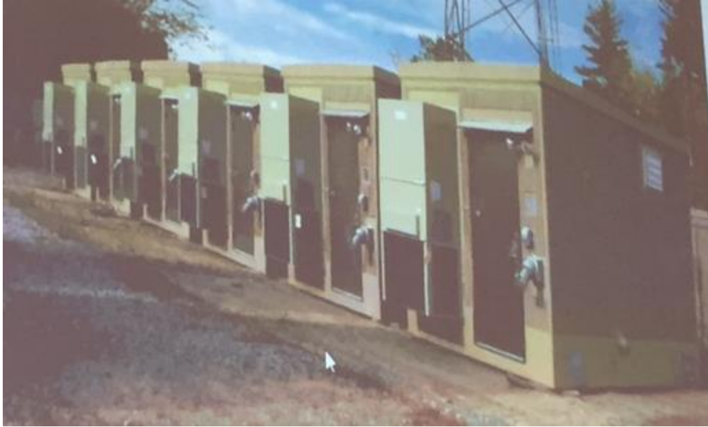
Comscope, 288 fiber panel Built up but left room for spare fiber; splitter chase with spacer plates Parking lot- port efficiency. 256 homes served- splitter tails available to other residents.
