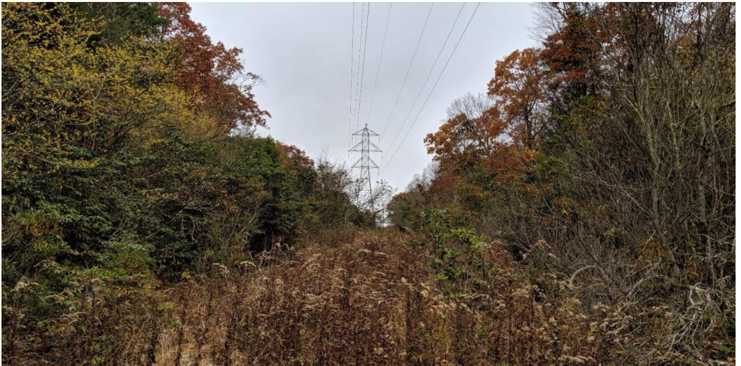
Photo #2: View of existing Structure 443 located within BVW SHU-W3A . Boring B-443 is proposed approximately 18 feet northeast of the existing structure and is located within the 100-foot Buffer Zone and Riverfront Area. Temporary construction matting in BVW SHU-W3A is required in order to access B-443. Facing northwest.
