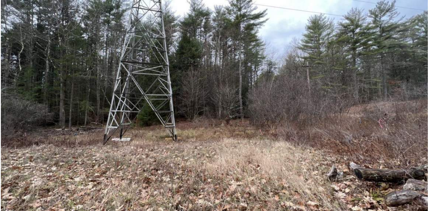
Photo #1: View of existing Structure 436 located within BVW SHU-W5. Boring B-436 is proposed approximately 18 feet southeast of the existing structure. Temporary construction matting in BVW is required in order to access and create a workpad for the work. Facing southwest.
