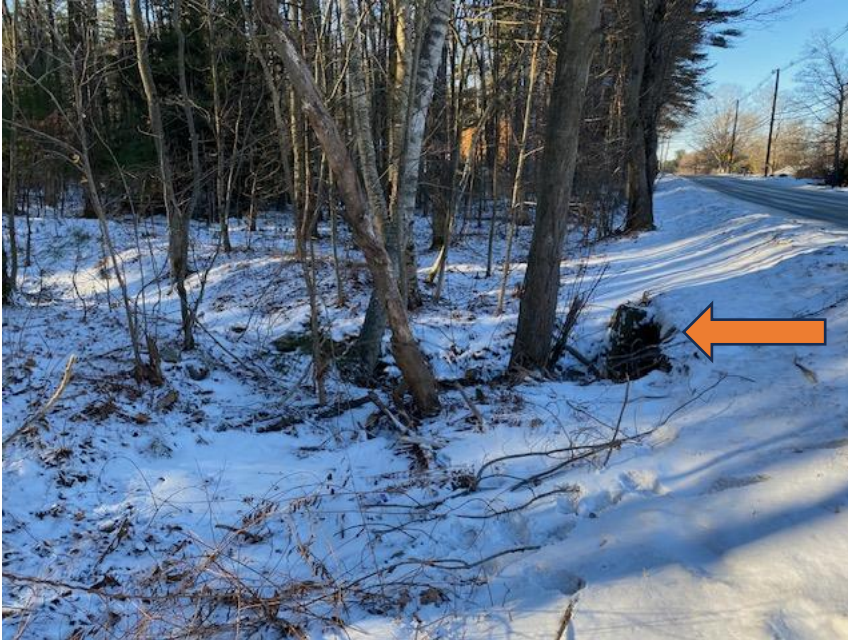
Photo 5 - Photo of culvert inlet on Leverett Road
