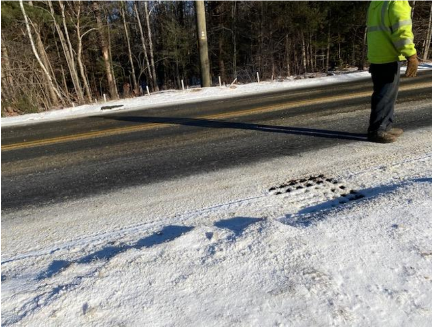
Photo 1 - Grate in Leverett Road
