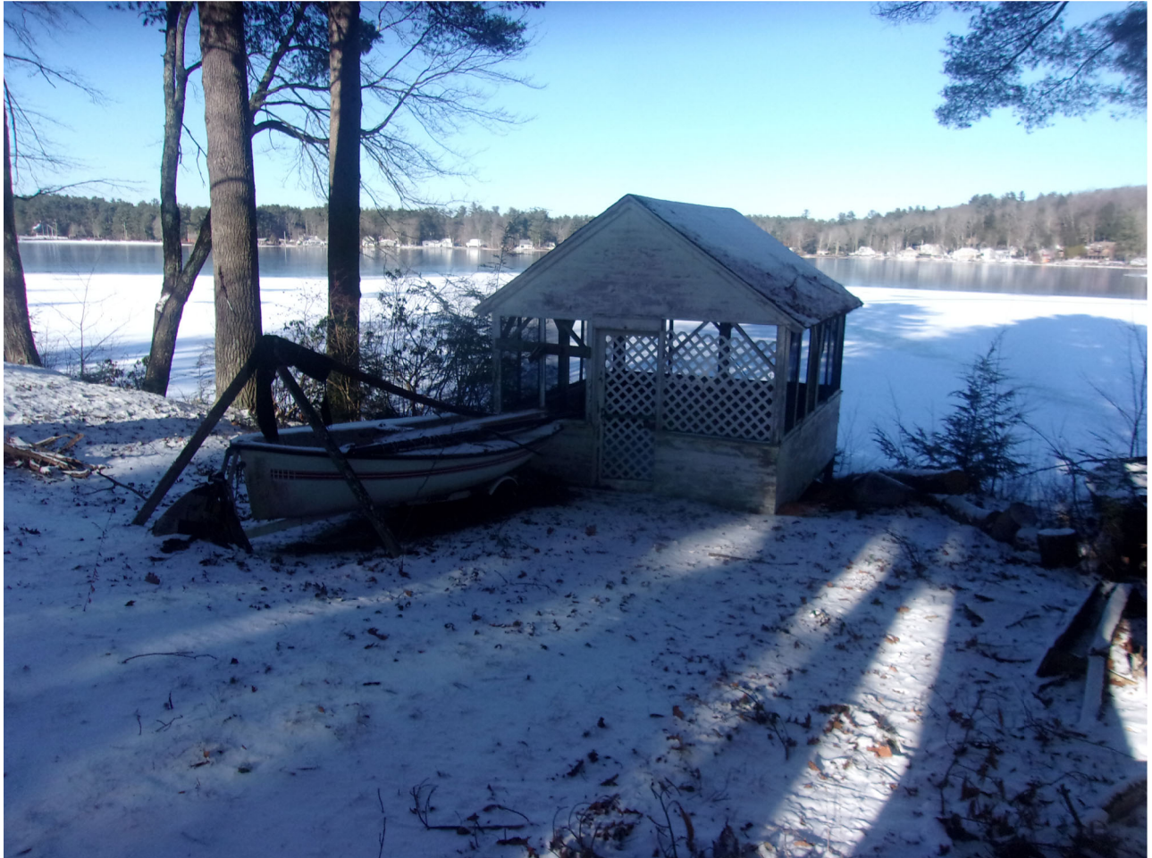
Photo 4 - existing boathouse to be renovated. Dock will be placed to the left of trees in picture.
