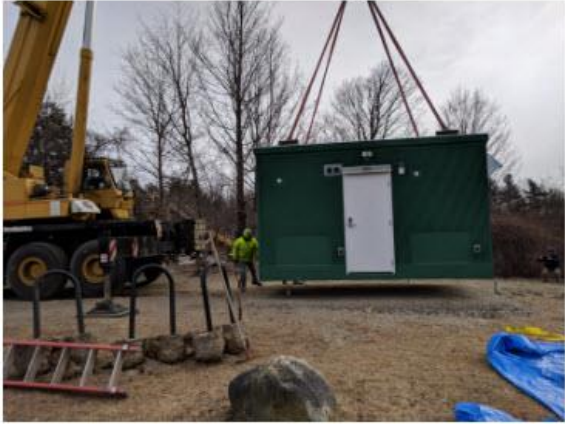
The hut arriving and being lowered into place
