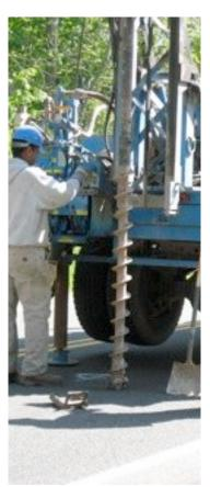
The crew from Seaboard Drilling Company worked with our environmental scientist, Joel Harris, to take numerous samples at different depth. We were surprised to be able to drill to 14' without hitting any bedrock. We hit bedrock at 2 other locations during the big dig and there have been many stories of bedrock being hit over the years and during the LCP road project. Five samples were taken and did prove to show contamination at 6-8'.
