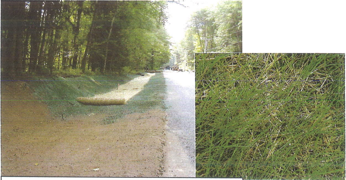
Figure 12 Turf Reinforced Mat Placement on Route 32A in Hardwick, MA. (DCR/DWSP)
