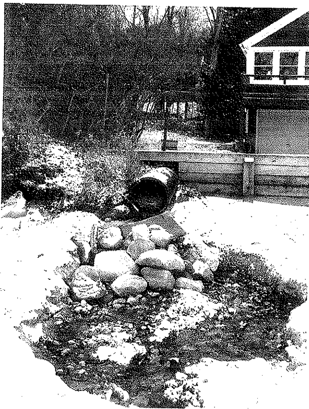
Figure 4B Storm drain outlet on shore of Lake Wyola. (DCR/DWSP)
