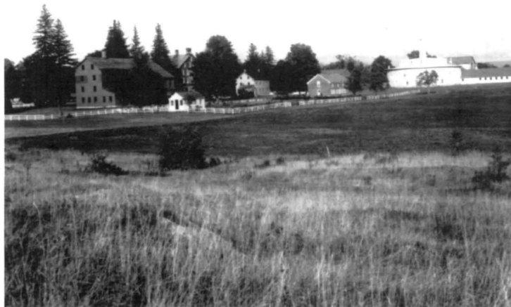
The fact that a property has religious connotations does not automatically disqualify it for inclusion in the National Register. This Shaker community in Massachusetts, for example, while religious in orientation, is included in the Register because it expresses the cultural values of the Shakers as a society. (Historic American Buildings Survey)
