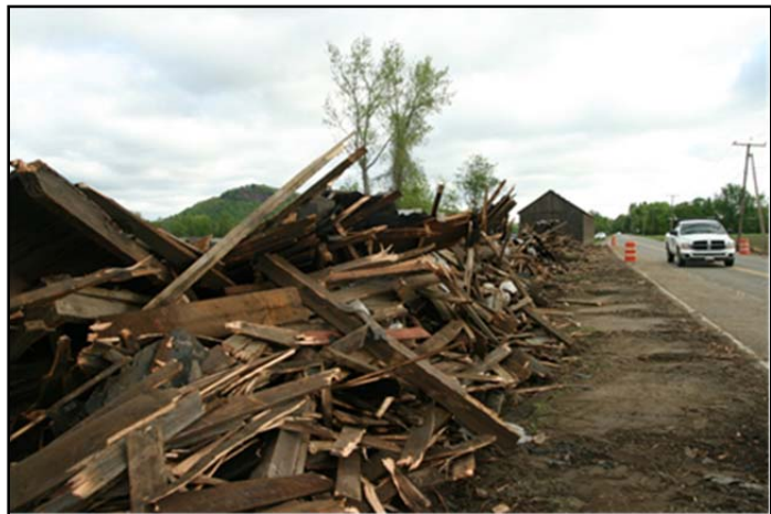
The aftermath of the gustnado that destroyed this Sunderland barn in 2009.
