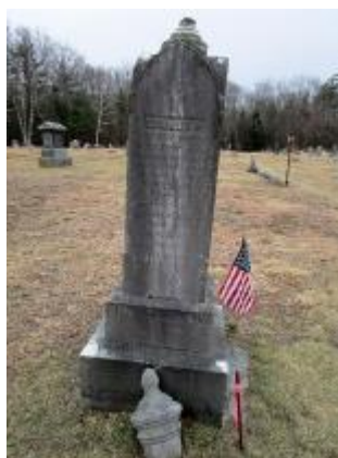
E.P. Pierce monument needing repair and cleaning.
