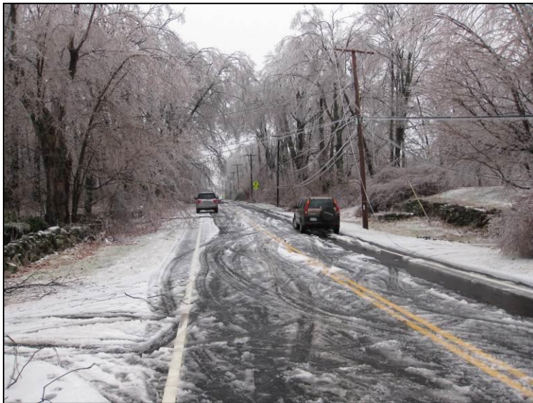
Ice covered trees and roads in Shutesbury after 2008 ice storm
